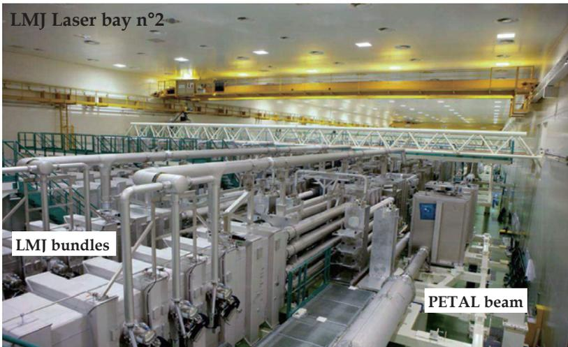
Figure 1: One of the four LMJ laser bays with 7 LMJ bundles (56 beams) and PETAL beam
